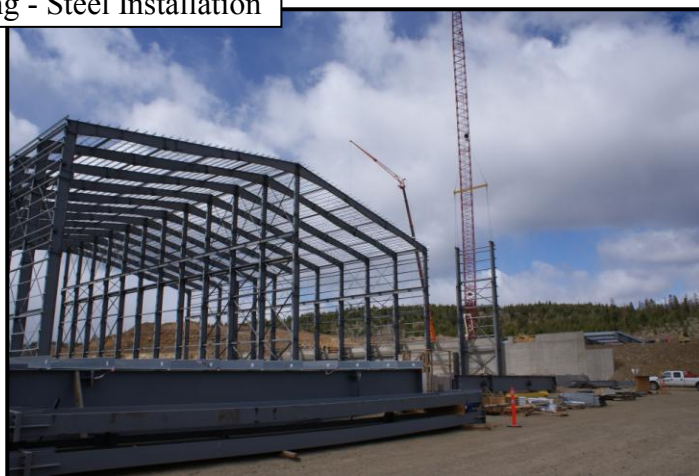
Concentrator Building - Steel Installation
