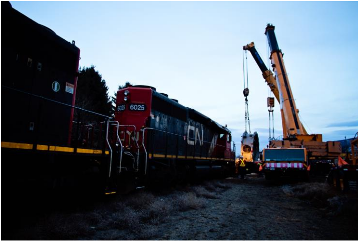
Unloading of lower bowl assembly in Kamloops, BC
