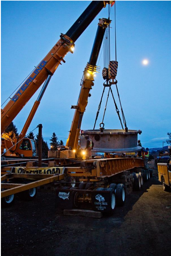
Placement of lower bowl assembly on transport trailer
