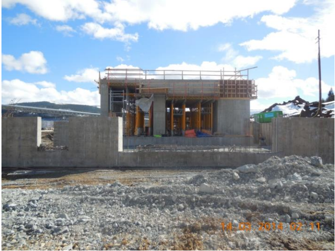
North side of secondary crusher foundation work at mine site
