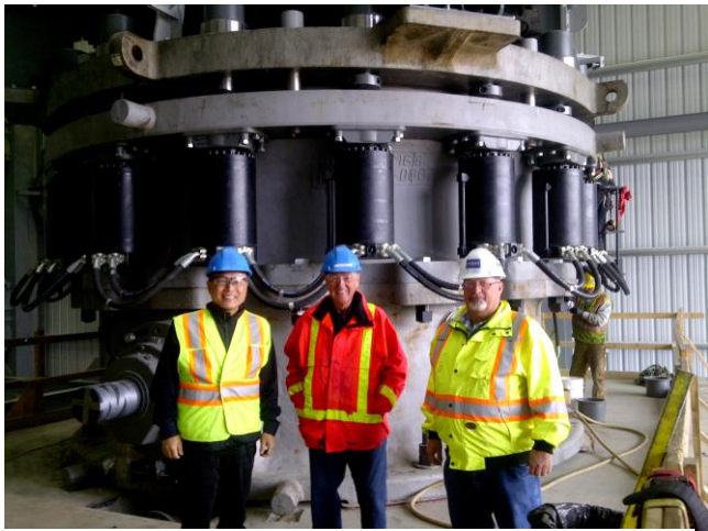
Lower and Upper Main Frames installed
