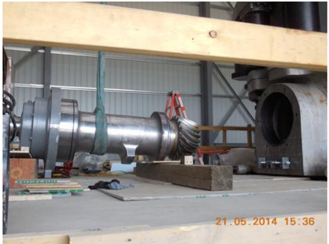
Prepping countershaft for installation
